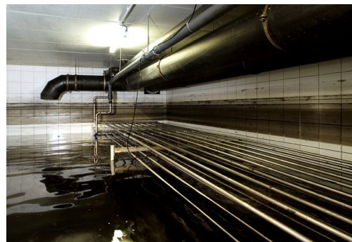
Absorber in the settling basin with lowered water level
