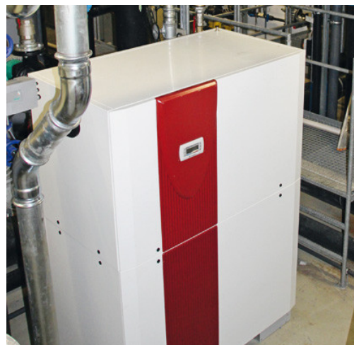
One of two water-to-water heat pumps Dimplex model WI 100TU
