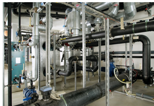
Transfer station for heating the indoor and outdoor pools
